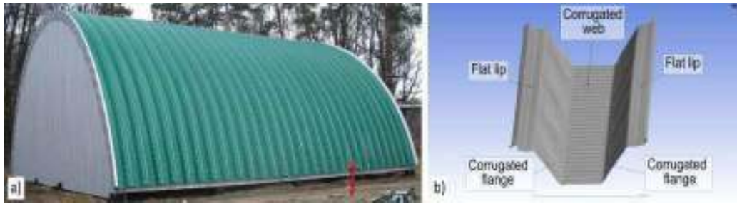
Figure 1. (a) Outside image of the measured hall as an example of typical self-supporting arch-shaped covering, (b) section surfaces.
